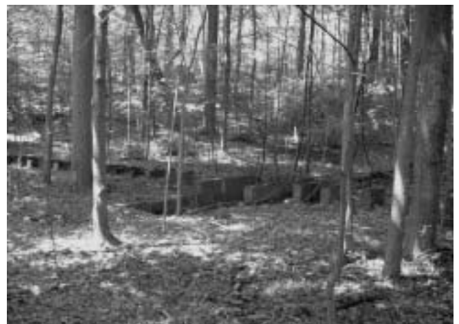
Remains of Long Pond sawmill, west of Long House Road..
